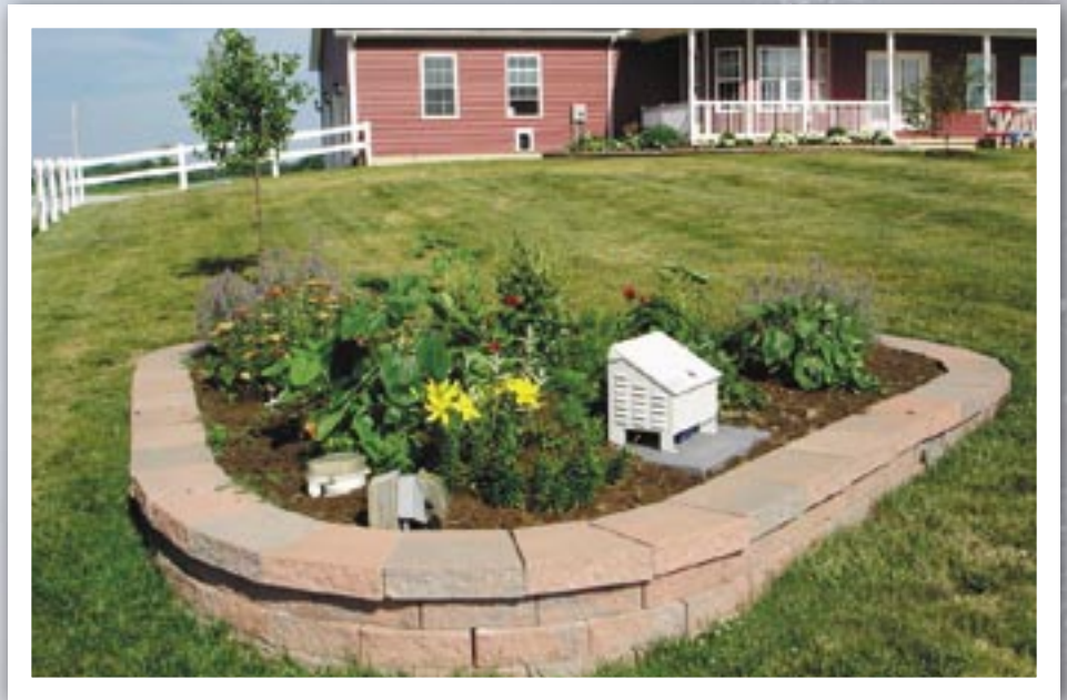
The air compressor box can be thoughtfully placed, out of the way and unobtrusive.
