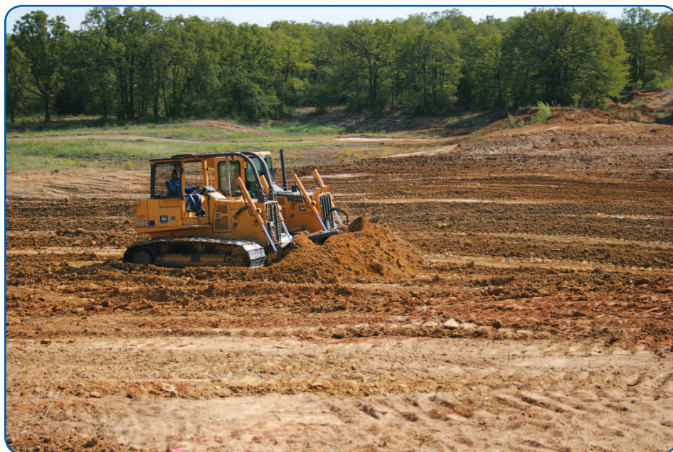
Droughts are often the best times to renovate. Here, Mike Otto is removing bottom soils from an older pond to deepen and widen it for the landowner.
